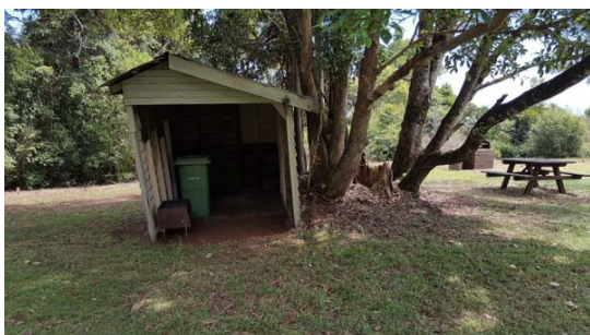
The 'lean to' shed emptied, cleaned and trees pruned
