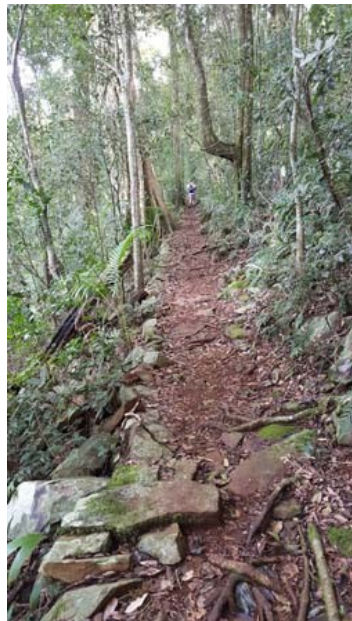
Repairs to the track footing
