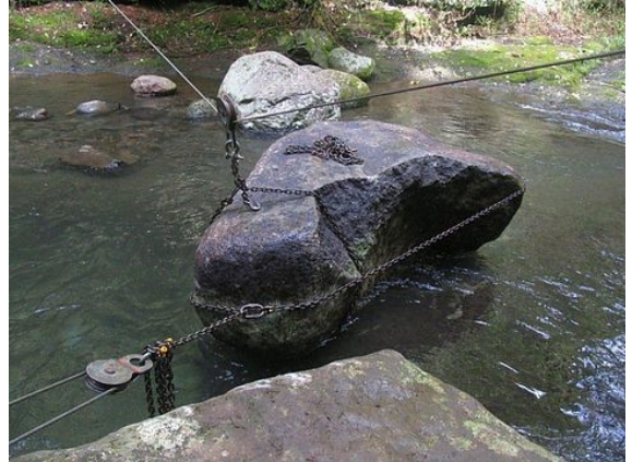
Box Forest Track repairs at Lamington NP
